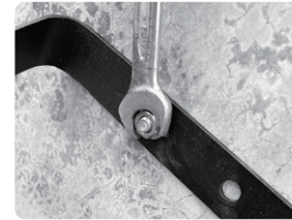
7. Tighten the two nuts with wrench.
