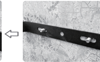
5. Place the light bracket over the fixings.
