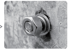
3. Place the expansion screw into the hole.
