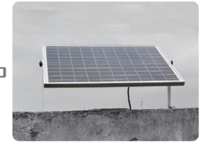
10. Install the solar panels in the location, and make sure solar panel is exposed to full sunlight.
